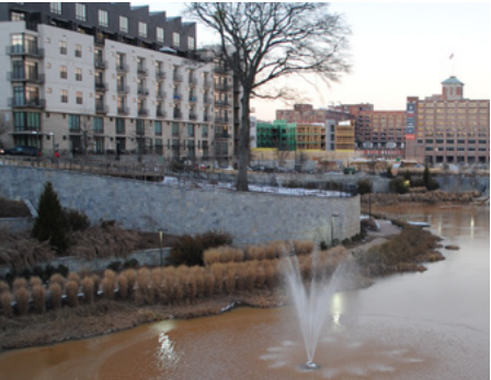
Providing detention/retention features within landscapes will allow water to percolate naturally over longer periods. When not filled with water, these can serve as both open and functional spaces.
