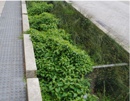
Features like bioretention basins along roadways can help slow water down in larger rain events by creating small pools with weirs, which overflow to the larger system.
