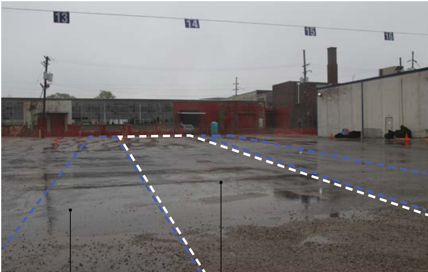
Excess parking spots can be removed and regraded as bioswales to clean and soak up runoff from the parking lot.
