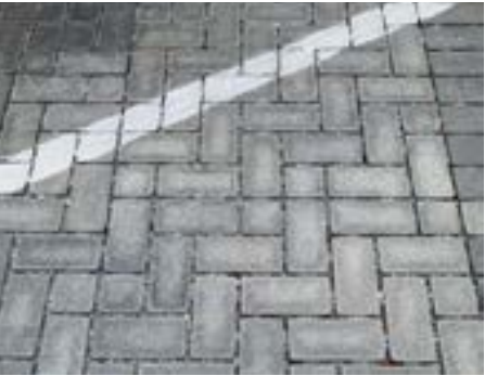
Pervious surface materials that allow the landscape to act more like a sponge, such as the materials used in this parking lot, can dramatically reduce runoff.
