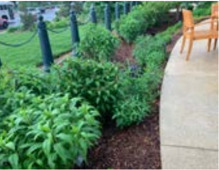
Using topography like this designed basin will help capture and slow stormwater runoff while improving a community streetscape.
