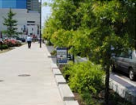
Linking stormwater collection points along green streets can create networks of stormwater features, providing multiple benefits to both the streetscape and the stormwater collection system.
