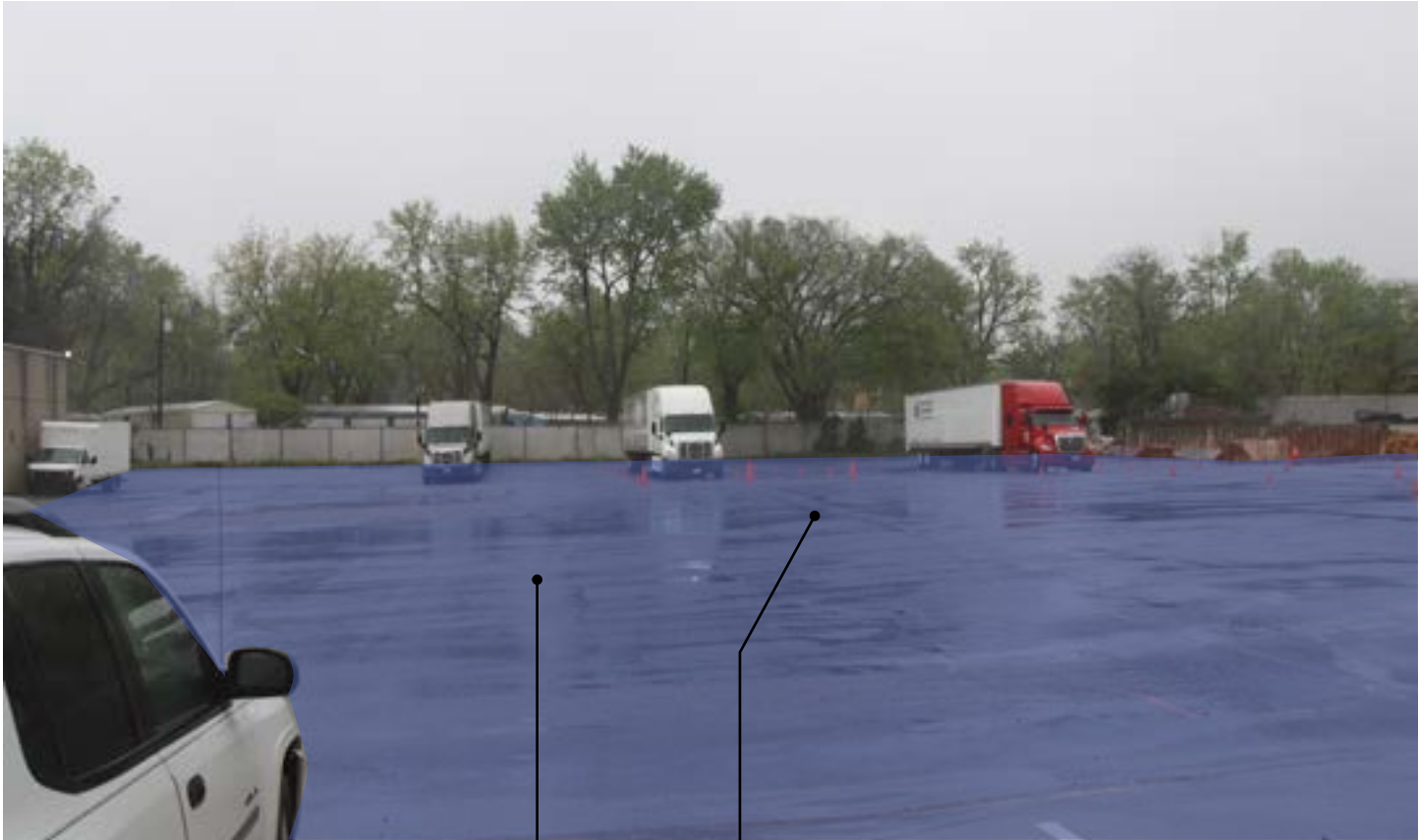
As the site exists, during rain events, water ponds in low spots and creates standing water on the impervious surface.
