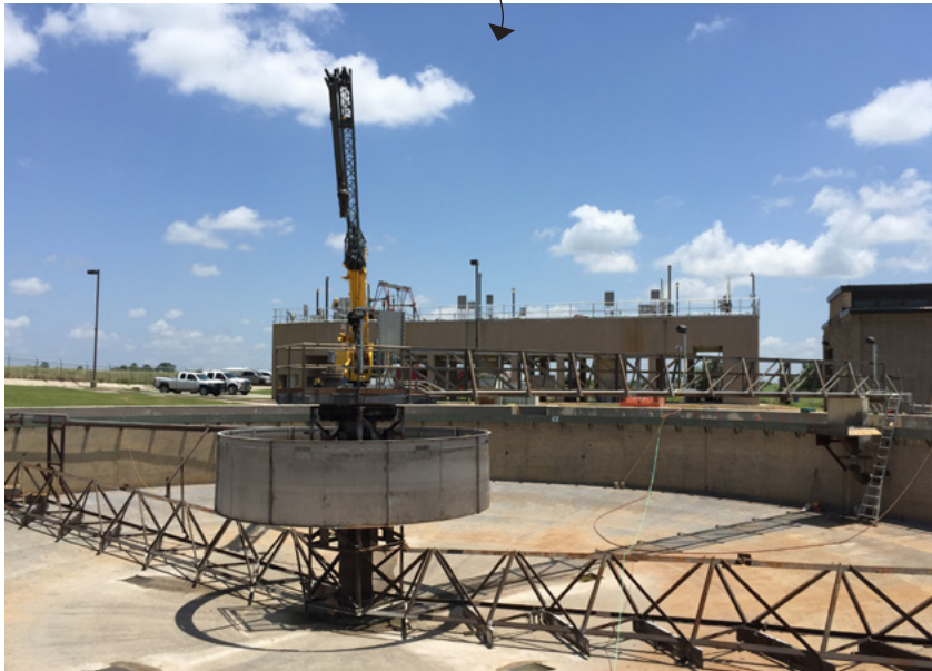
The clarifiers' concrete walls received a much-needed upgrade.
